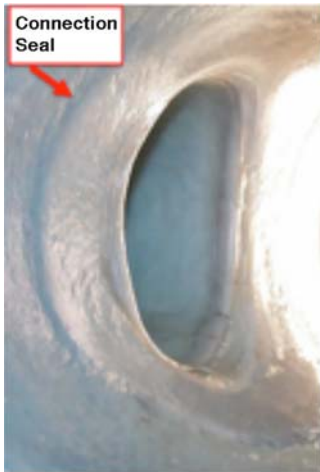
FIG. 5 SMHG Connection Seal after CIPP Installation
