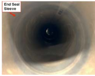
FIG. 4 SMHG End Seal after CIPP Installation
