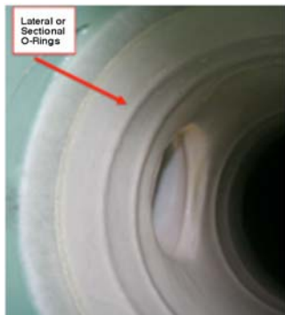
FIG. 6 SNHG O-ring after CIPPP Installation
